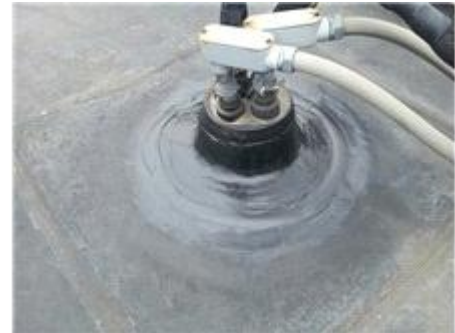
03R - Portal Repaired Areas:1
