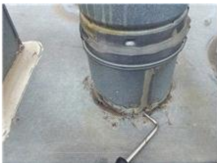
Copy Of 12 - Flue Pipe Before
