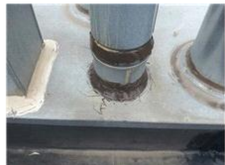
12R - Flue Pipe Repaired Areas:2
